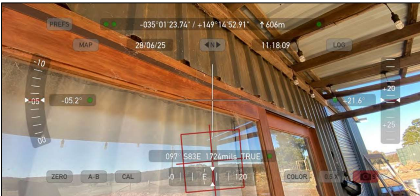
Photo point 14 Looking at example of glazed element (note no flyscreens and example of gaps at intersection of cladding and timber framing. (TANX Environmental, 2025)
